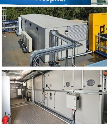
Our team worked closely with Lewisham and Greenwich NHS Trust's M&E Services Contractor to design and supply this bespoke supply & extract heat recovery AHU c/w reverse cycle direct expansion (DX) coil, and energyefficient EC plug fans.
