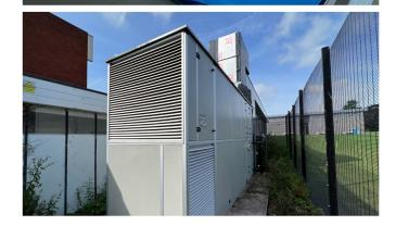
To assist in reducing running costs, AirCraft Air Handling manufactured an efficiency heat recovery AHU incorporating a plate recuperator that offers c.75% reduction in heating costs vs the original AHU, along with high-efficiency EC fans that save on electrical running costs and lowering maintenance costs by omitting the traditional belt driven fans of the old unit.
