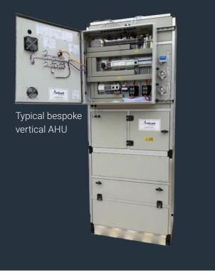
AHU system capable of filtering, recirculating, cooling and heating the air within the new main shopping mall area. Due to the size of the shopping mall, AirCraft Handling manufactured twelve vertical AHU units.
