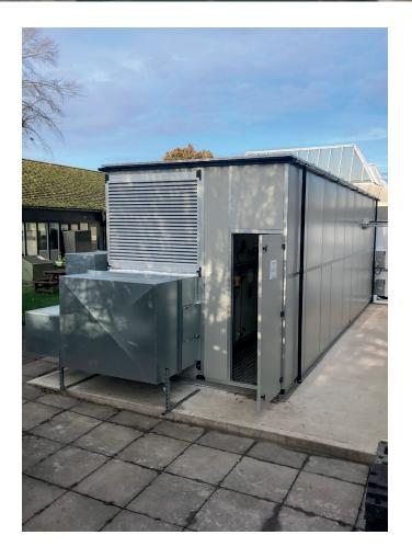
Working with our customer, AirCraft Air Handling's designers and technical engineers proposed that we manufacture a self-contained AHU unit with a narrower service corridor of only 1200 mm wide. This would provide ample space for maintenance engineers to work within the enclosure.
