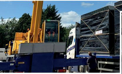
The AHU section would be designed at a maximum width of 1600 mm. The choice of components selected for the AHU needed to be small enough for maintenance engineers to easily withdraw them from the unit if repairs or replacements were required in the future. The combination of the overall dimension reduction of the self-contained plant room and its internal components collectively achieved the significant cost reductions the Trust was looking for.
