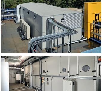
Our team worked closely with Lewisham and Greenwich NHS Trust's M&E Services Contractor to design and supply this bespoke supply & extract heat recovery AHU c/w reverse cycle direct expansion (DX) coil, and energyefficient EC plug fans.
